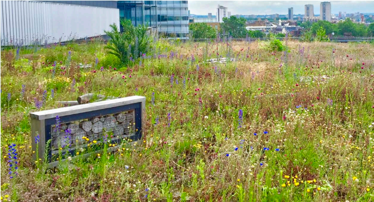
■ Green roof at PwC, London Bridge. Image source: Dusty Gedge, Living Roofs.
